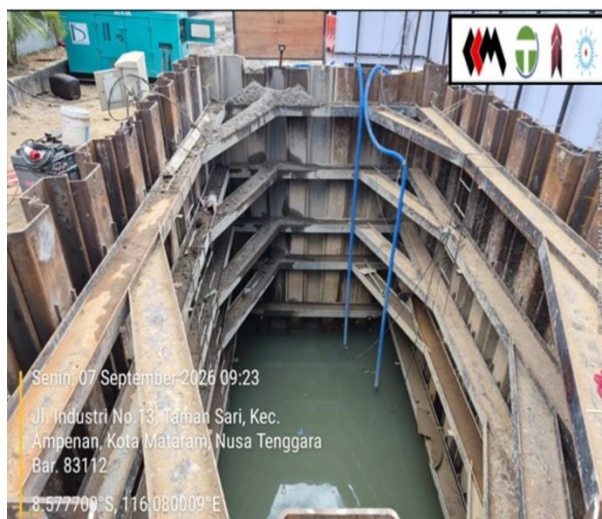
Gambar 4 Dewatering area galian
