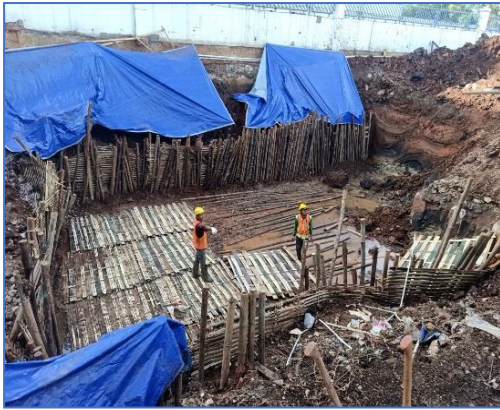
Gambar 7 Pasang Matras Bambu
